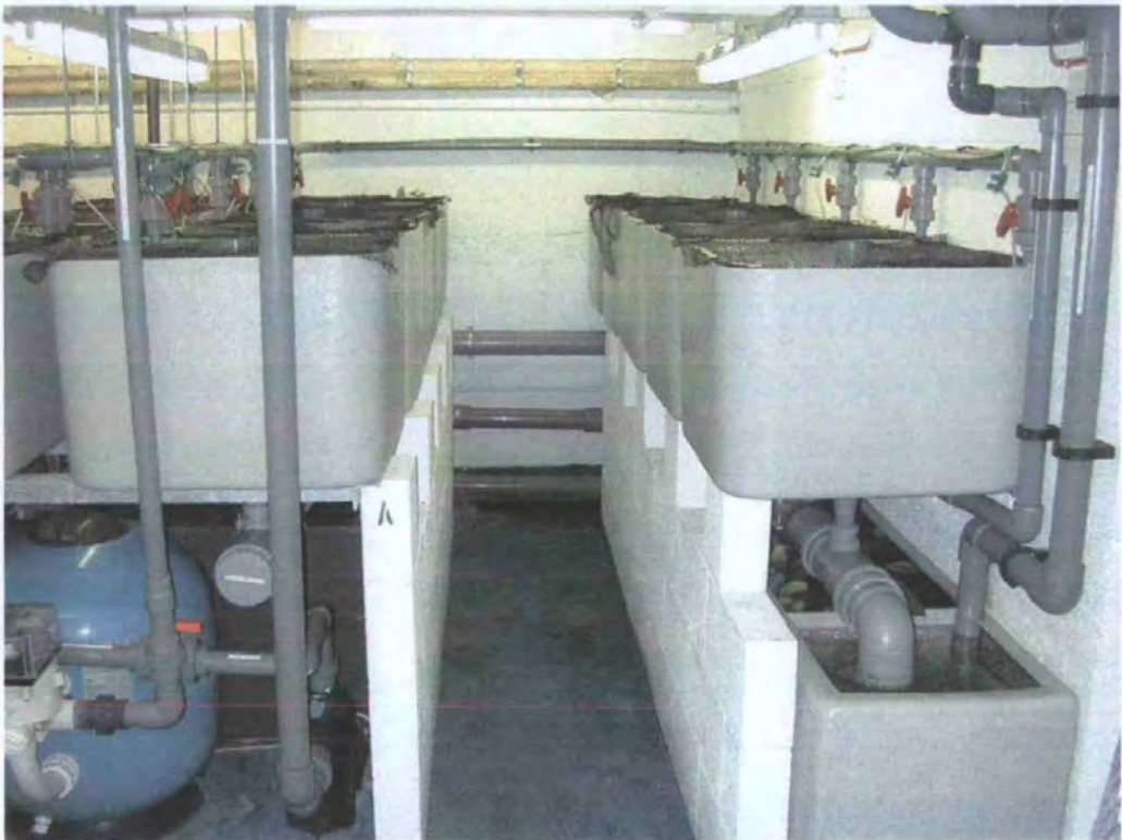
Figure 2.5 View of tanks 1-10 in aquarium system '1', sand filter (bottom left) and pre-filter tank (bottom right).
