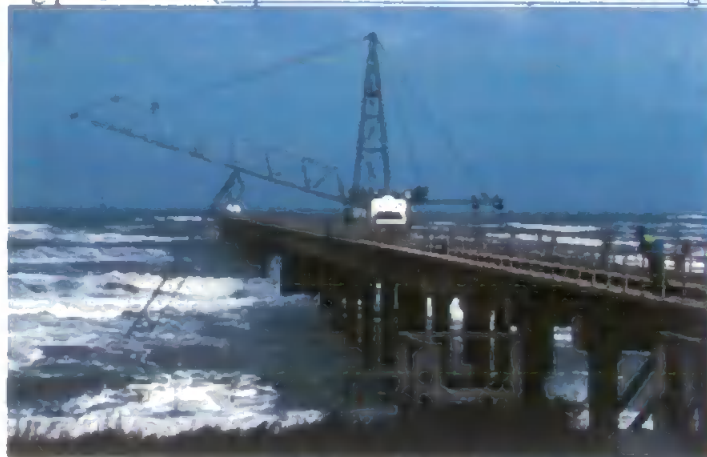
Sensor Insertion System at Duck ( http://www.frf.usace.army.mil/vehicles2.stm ).
