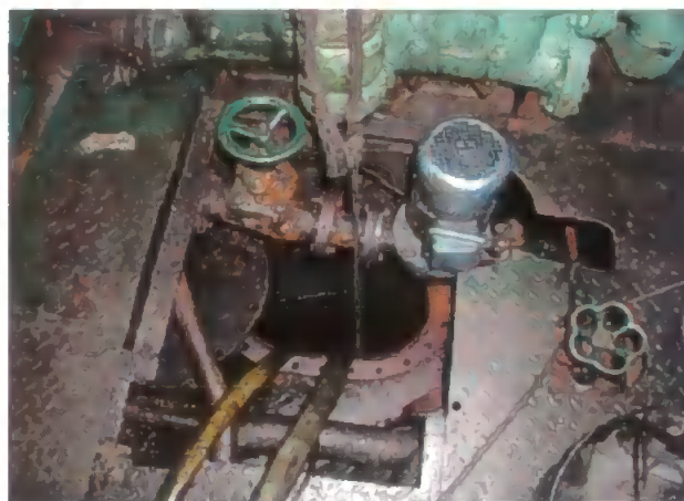
Fig. 5.6 Direct overboard bilge connection
