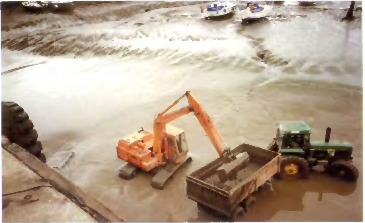
Figure 6-11 Dredging at Watchet at low tide
