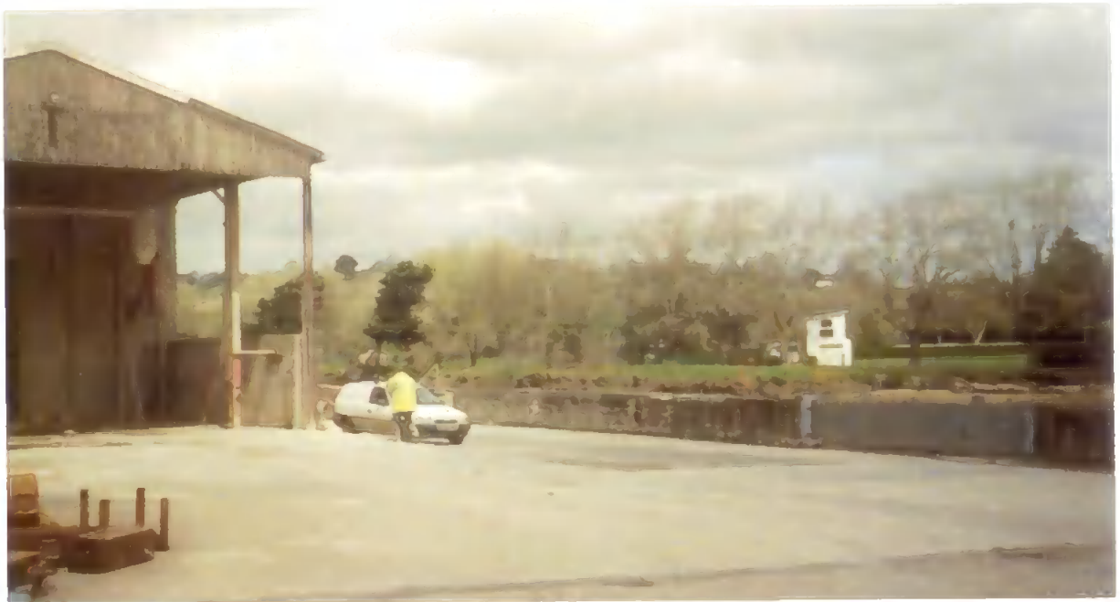
Figure 6-14 Lighterage Quay, Truro, showing the flood wall
