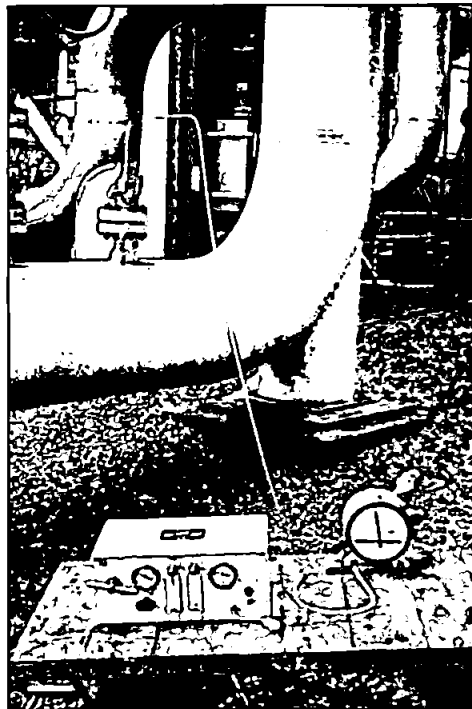
Figure 5.20. Connection of the sampling interface to the outlet pipeline of the mercury removal tower
