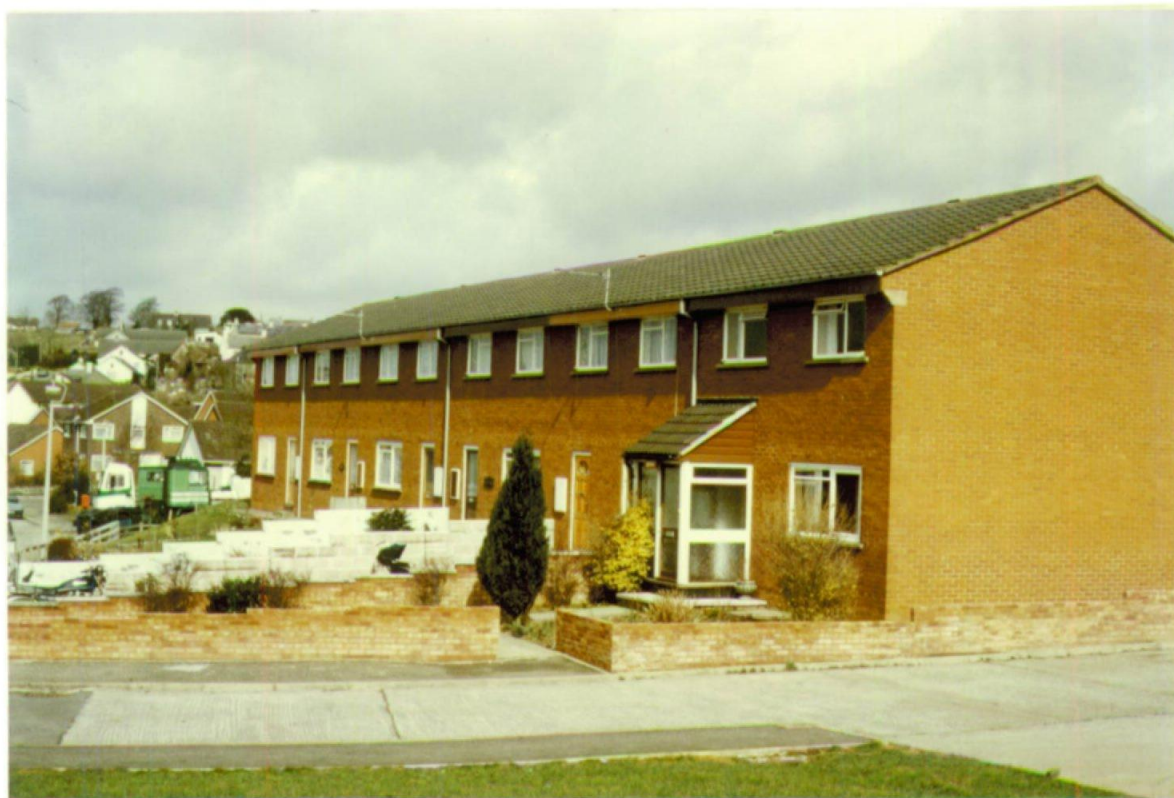
PLATE 3.12 THE SUCCESSFUL LOCAL AUTHORITY DEVELOPMENT AT CHURCHILL CRESENT, SOUTH MOLTON
