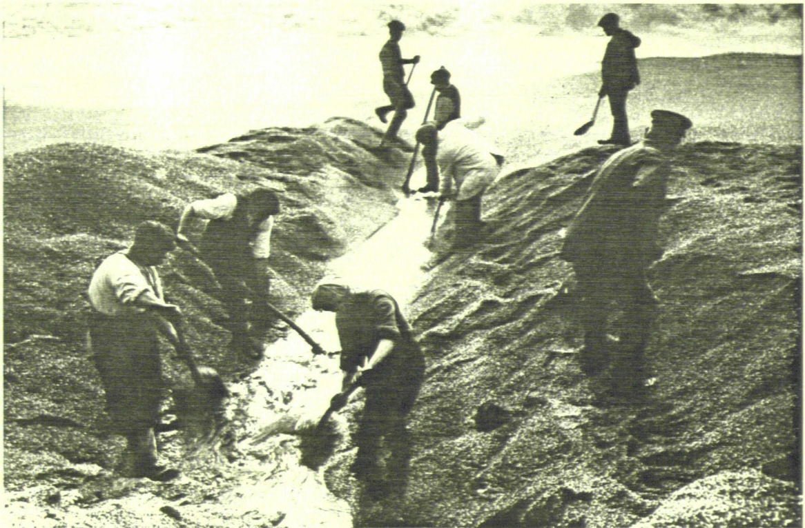
Plate 3.12: Clearing the outlet of the adit which had also been buried under large quantities of shingle. (From original photographs in Helston Folk Museum)
