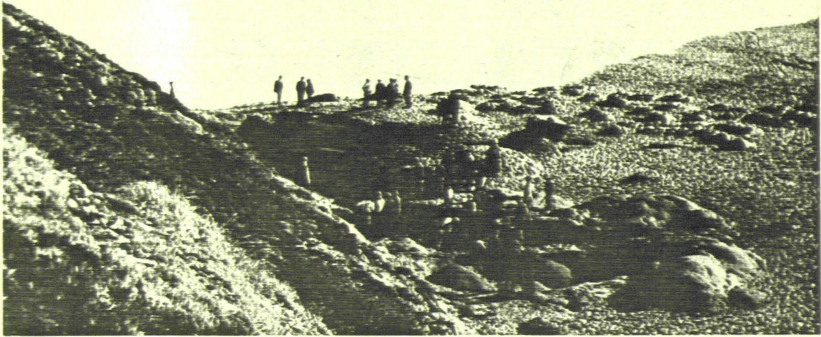
Plate 3.11: Clearing the mouth of the drainage adit in January 1924.
