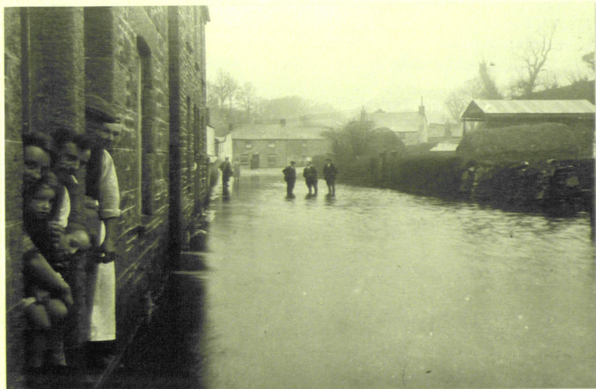
Plate 3.8: Lower Road in Helston, flooded in 1924 after the blockage of the Loe Pool drainage adit.
