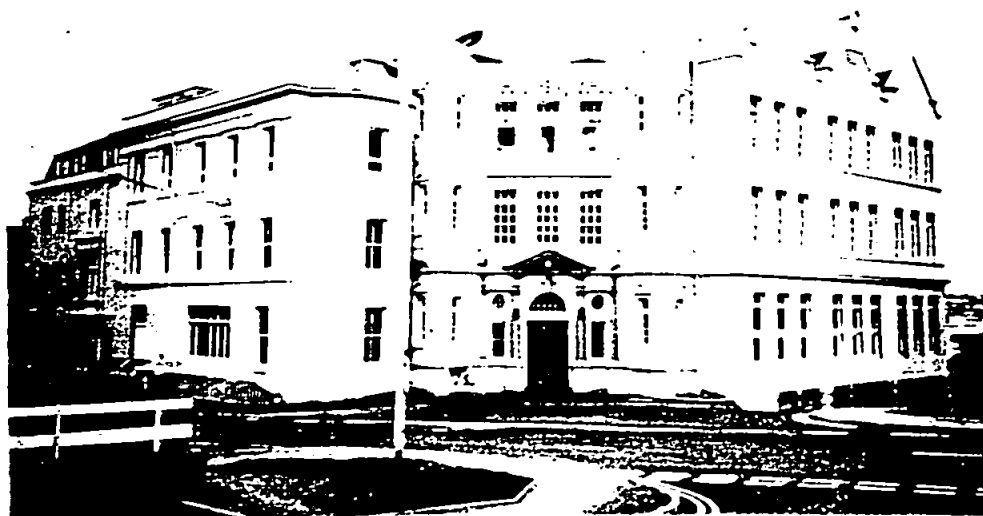
Devonport Royal Sailors' Home, now the Royal Fleet Club. This is the new building opened on 1902 in Morice Square, Devonport. Source: A photograph taken by the author, 1966.
