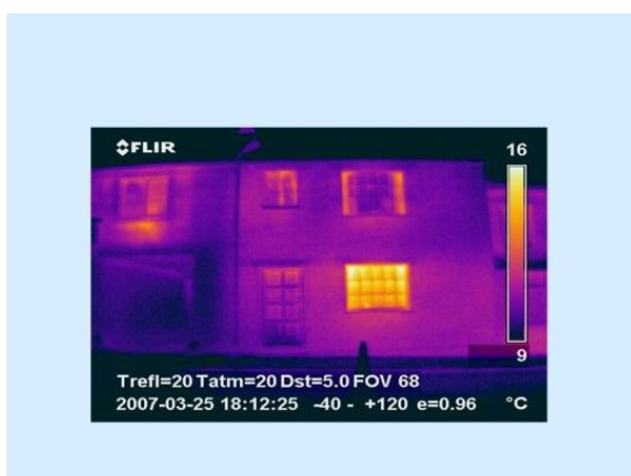
Figure 7.3: Thermal image showing a single glazed window.
