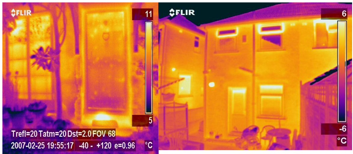
Figure 4.2: Thermal image example of two visible actions (draught proofing and closing windows when the heating is on).
