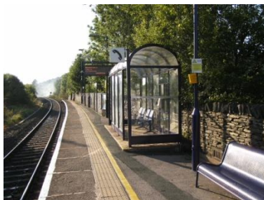
Staveley Station (No. 6 of 8)
