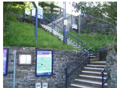
Staveley Station (No. 2 of 8)
