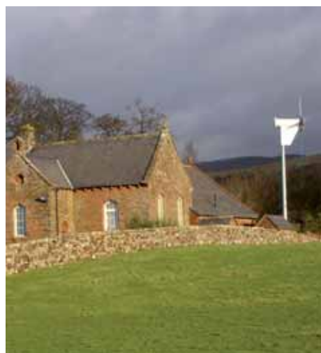
Gablesby village hall with its new turbine John Perkins
