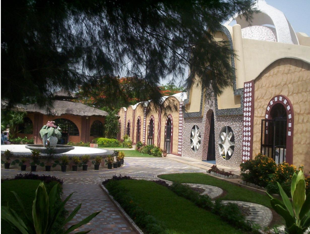
Figure 3.1: A school building designed and constructed by the author in Kaduna between 1997 and 2000. The author used CEB and also experimented on the use of adobe blocks with unstabilised earth rendering as well as the use of ferrocement and concrete on CEB walls and domes
