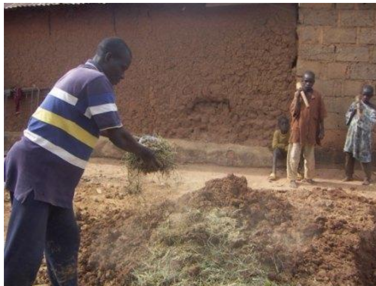
Figure 5.14: Straw is being added to wet soil mix
