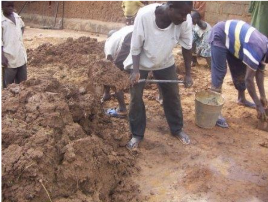
Figure 5.15: Final stage of soil mixing and moulding of adobe blocks
