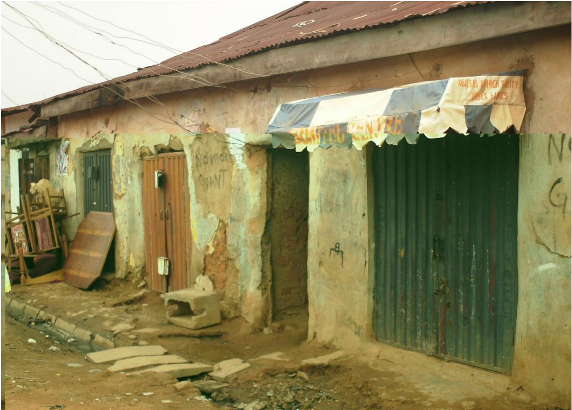
Figure 4.15: Adobe building with canopy, new doors, filled up window opening and new extension with lean-to roof at the far end
