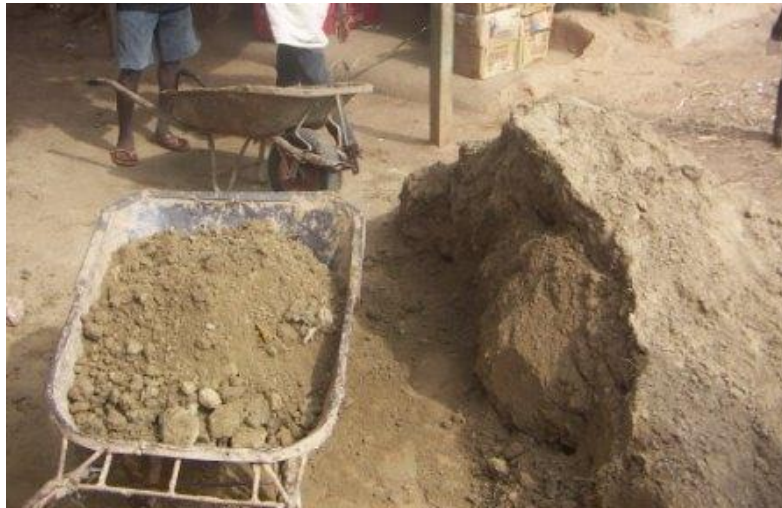
Figure 5.13: Crushed building earth ready for mixing
