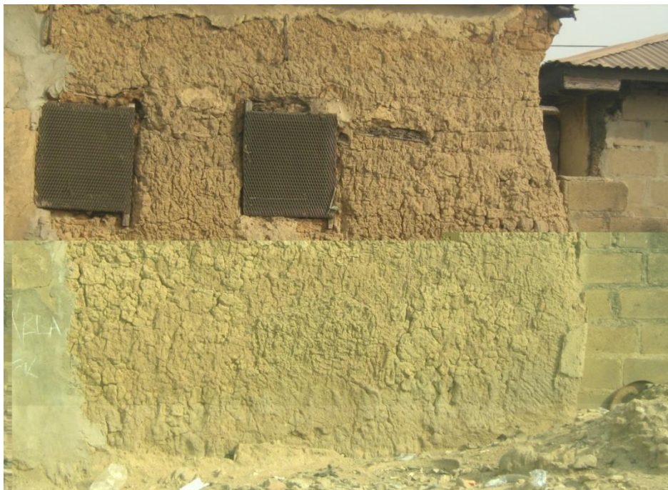
Figure 4.17: Adobe building with security screen on the windows
