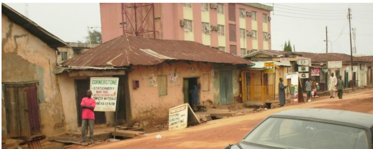
Figure 4.6: Single storey mix use adobe buildings behind a 4 storeys hotel constructed with concrete in Sabon Gari
