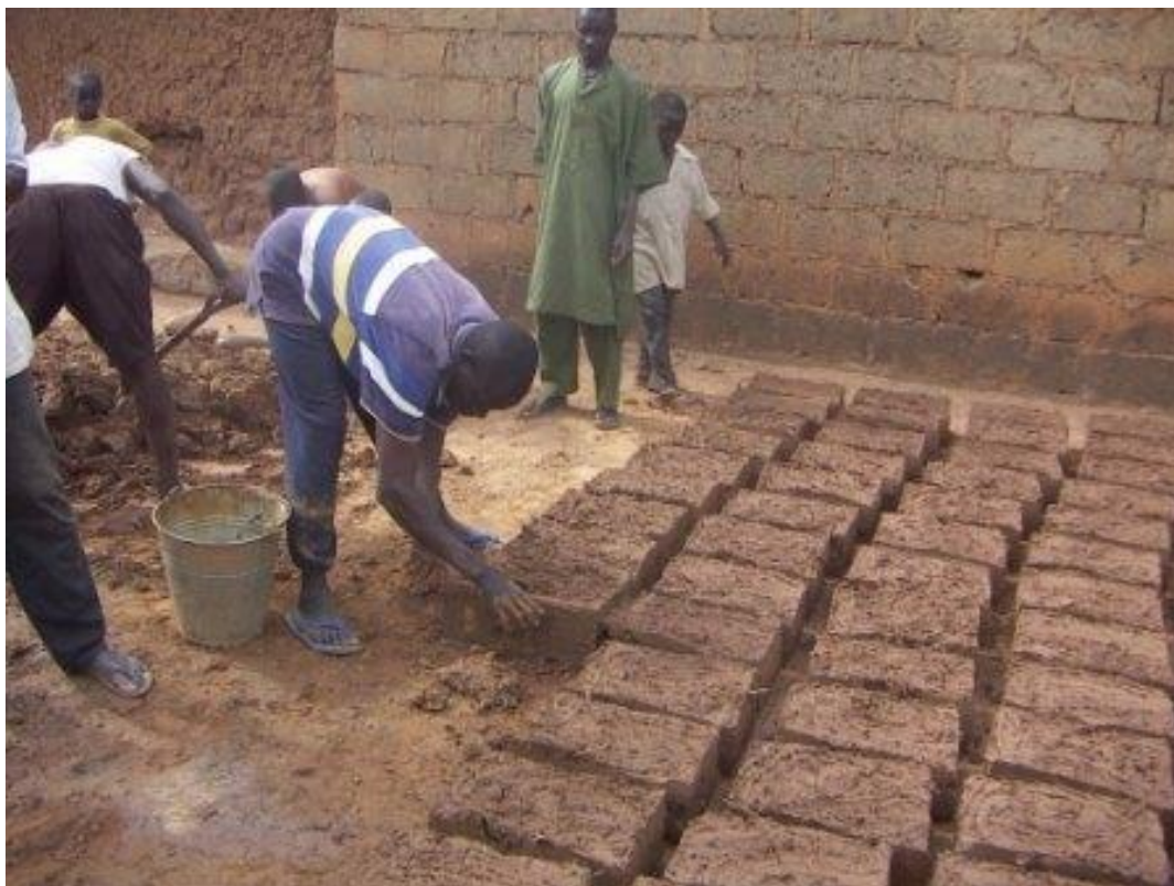
Figure 5.16: Demoulding of adobe block
