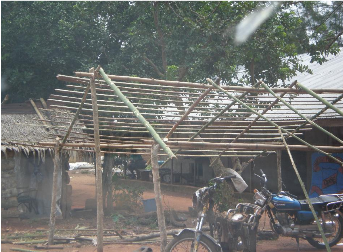
Figure 5.35: A wattle and daub building under construction
