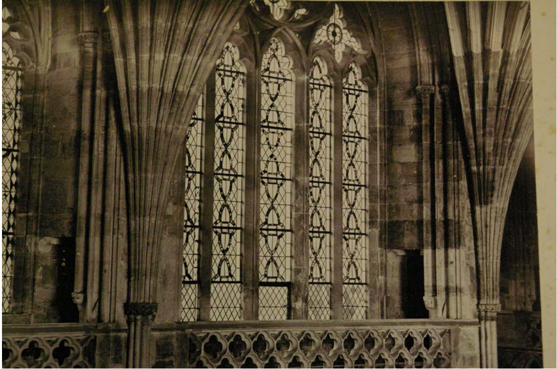
Figure 31: Sample of Glazing in the Clerestory circa 1903 showing the arrangement of mediaeval fragments in decorative medallions. Photo: Exeter Cathedral Archive. 1440-1444
