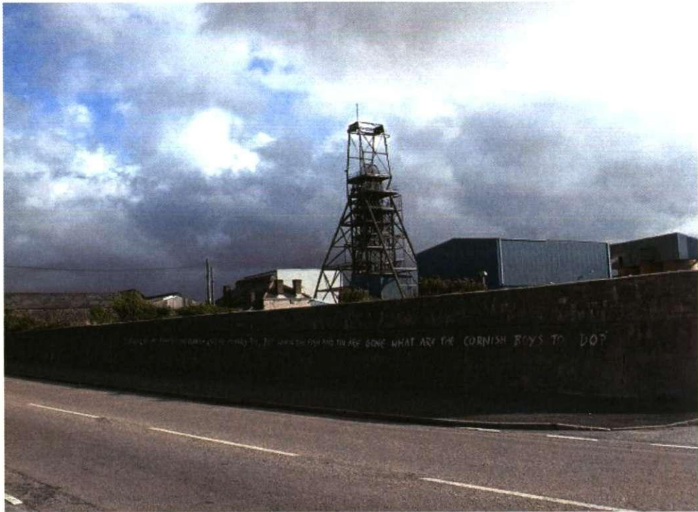
Figure 15: South Crofty Mine depicted after its closure in 1998.
