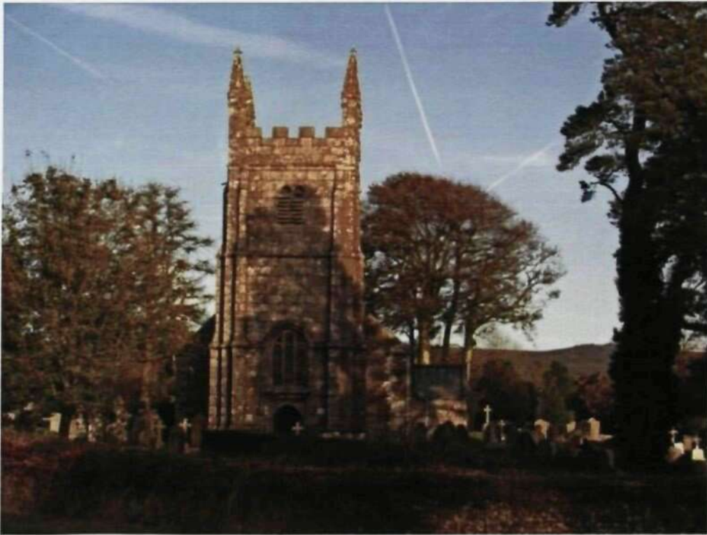
Figure 2.14 Lydford, Parish Church of St Petrock
