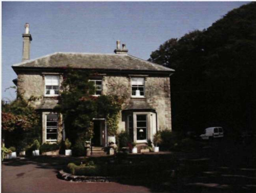
Figure 2.45 Tamar View (now know as the Horn of Plenty), near Tavistock, built by the Devon Great Consols Mine for its mine manager in 1866.
