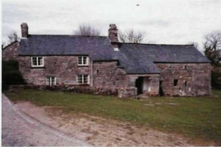
Figure 2.29 Sanders, Lettaford: a large, stone-built Dartmoor cross-passage longhouse which still has its large shippon intact.
