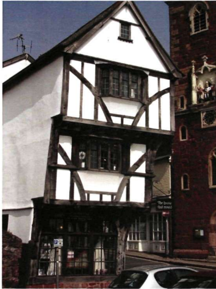
Figure 2.33 The 'House that Moved' at the foot of Stepcote Hill, Exeter. Threatened by demolition to allow for road improvements, it was moved on rollers to this position in 1961.
