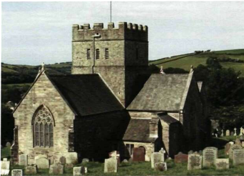
Figure 2.18 St Andrews Church Aveton Giffard. The original church comprised a cruciform medieval structure until it was heavily damaged by bombing in the Second World War. The church was rebuilt as a copy of the medieval original but has additional heritage significance as a result of its wartime damage and post-war restoration.
