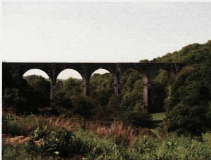
Figure 2.58 Derriton Viaduct, Holsworthy, completed in 1898 and restored as a footpath and cycle track with Heritage Lottery Fund support in 2007.
