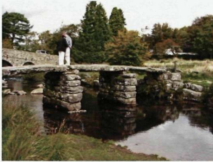
Figure 2.56 Postbridge, Dartmoor Clapper Bridge.
