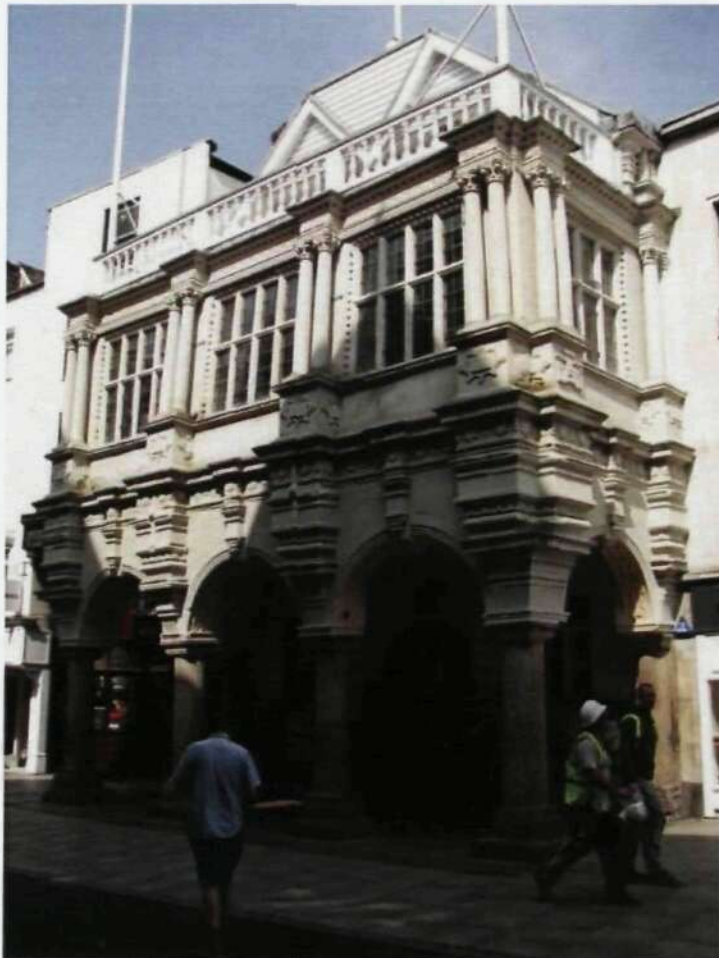
Figure 2.32 The Guildhall, Exeter. The original medieval structure was rebuilt in the 1590s.
