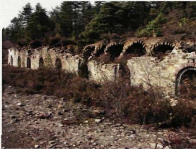
Figure 2.54 Remains of an Arsenic Calciner, Blanchdown Woods, Tavistock. This is an area of toxic ground and other hazards.
