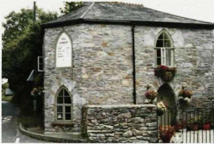
Figure 2.57 Former Turnpike Tollhouse (on A379), now used as private house, but displaying board showing charges or tolls for users of the thoroughfare in the turnpike era.
