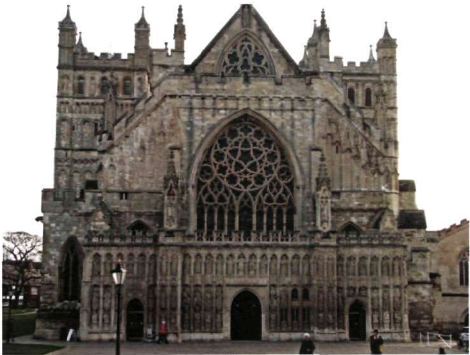
Figure 2.16 Exeter Cathedral, displaying Romanesque, Early Gothic, Decorated and Perpendicular architectural elements.
