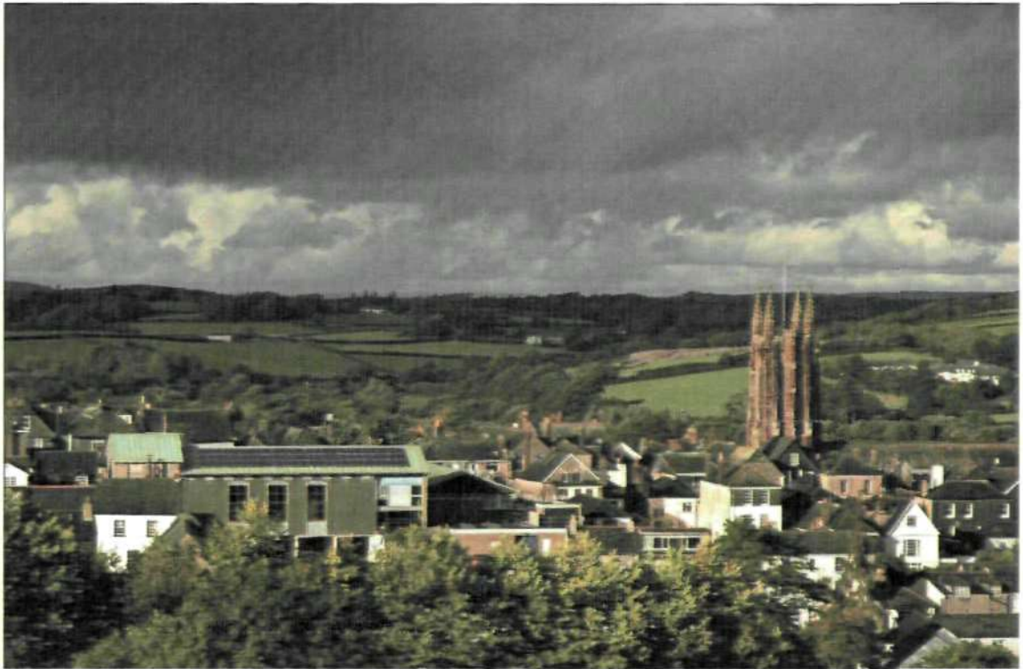
Figure 7.6. Panorama of Totnes town showing the Civic Hall with its new photovoltaic roof installed as part of the Transition Streets initiative (Source: Lou Brown/Transition Streets).
