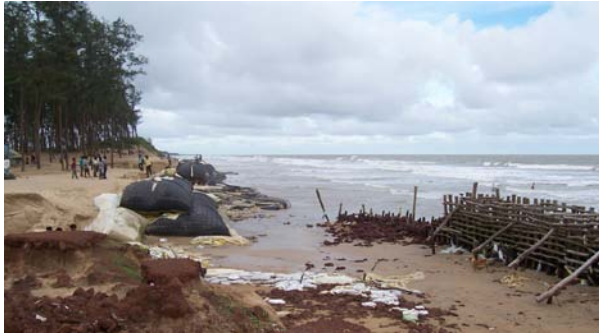
Fig. 7— Effect of surge on Geo-tube in Zone II
