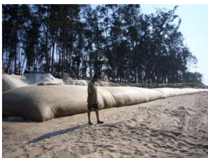
Figure 6- Geo-tube being constructed along the coastal stretch of Risk Zone II
