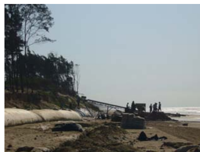
Figure 6- Geo-tube being constructed along the coastal stretch of Risk Zone II
