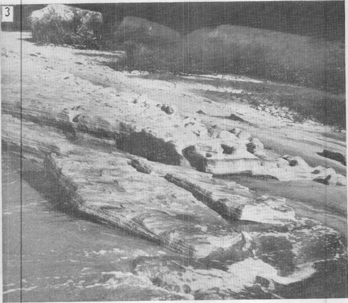
Fig. 3 — Hardened beach rock at Sethukarai (Rock is undercut by erosion and large blocks break and fall apart)
