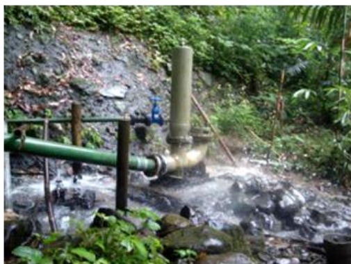
Gambar 2. Operasi pompa hydram
