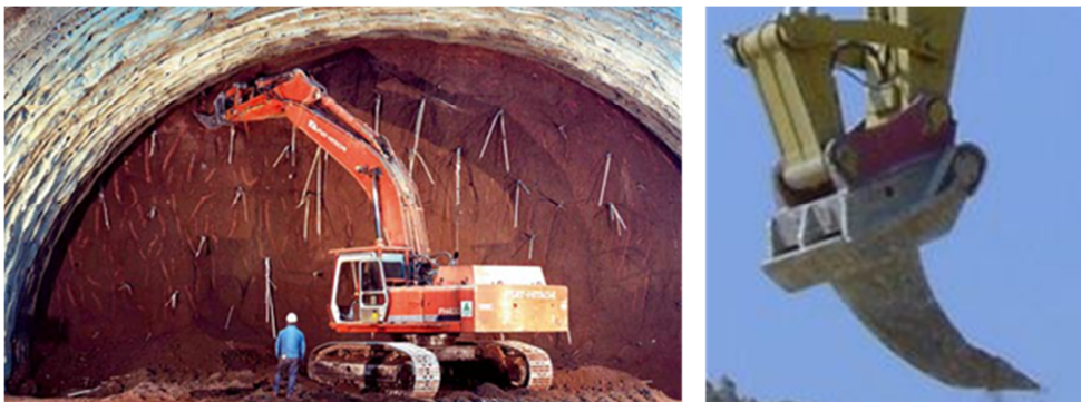
Figure 6. Crawler excavator equipped with ripper
