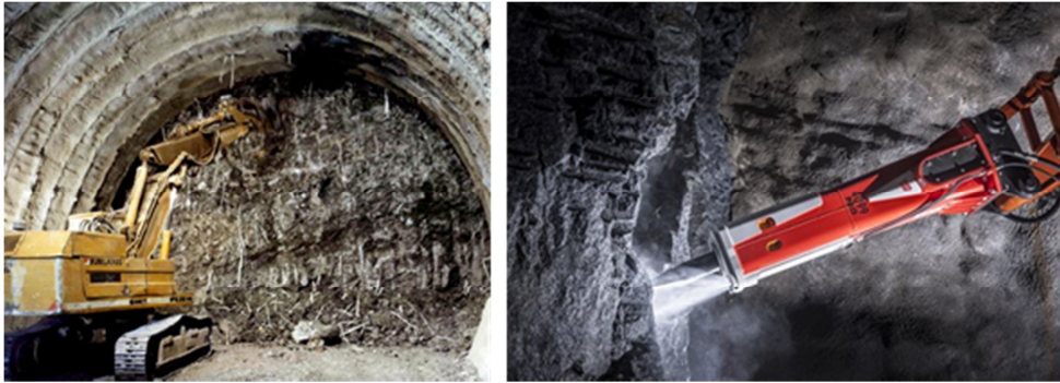
Figure 5. Crawler excavator equipped with hammer
