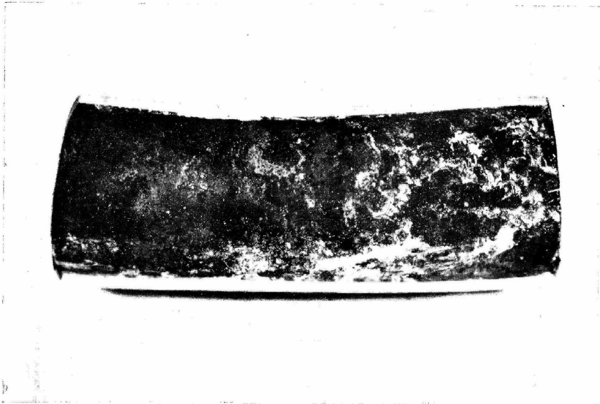
Fig. 10. Localized corrosion attack due to high concentration of dissolved oxygen
