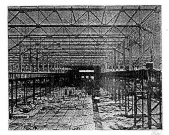
7 Building erection, plant installation, and plant foundation being carried out concurrently. Building is complete at far end of bay; EOT crane installed
