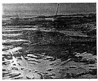
4 Early stages of site levelling. Up to 10m.yd<sup>3</sup> of spoil may have to be removed
