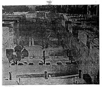
8 Mill foundations being prepared to receive the stands. Levelling pads being grouted in foreground
