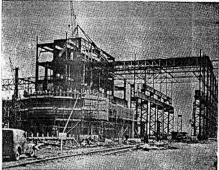
6 LD converter building during construction. Supporting structure for the vessel is being erected concurrently with the building
