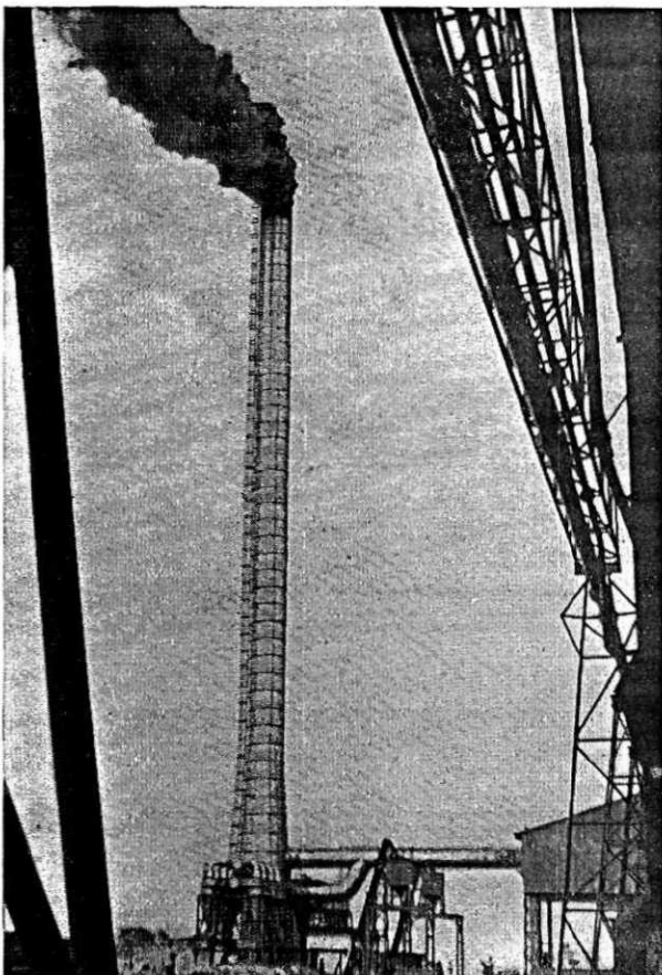
4 Chimney emitting dense brown fume during desiliconizing
