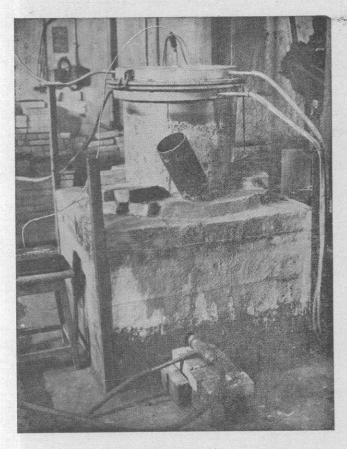
2 Photograph of the vacuum zinc distillation unit in operation
