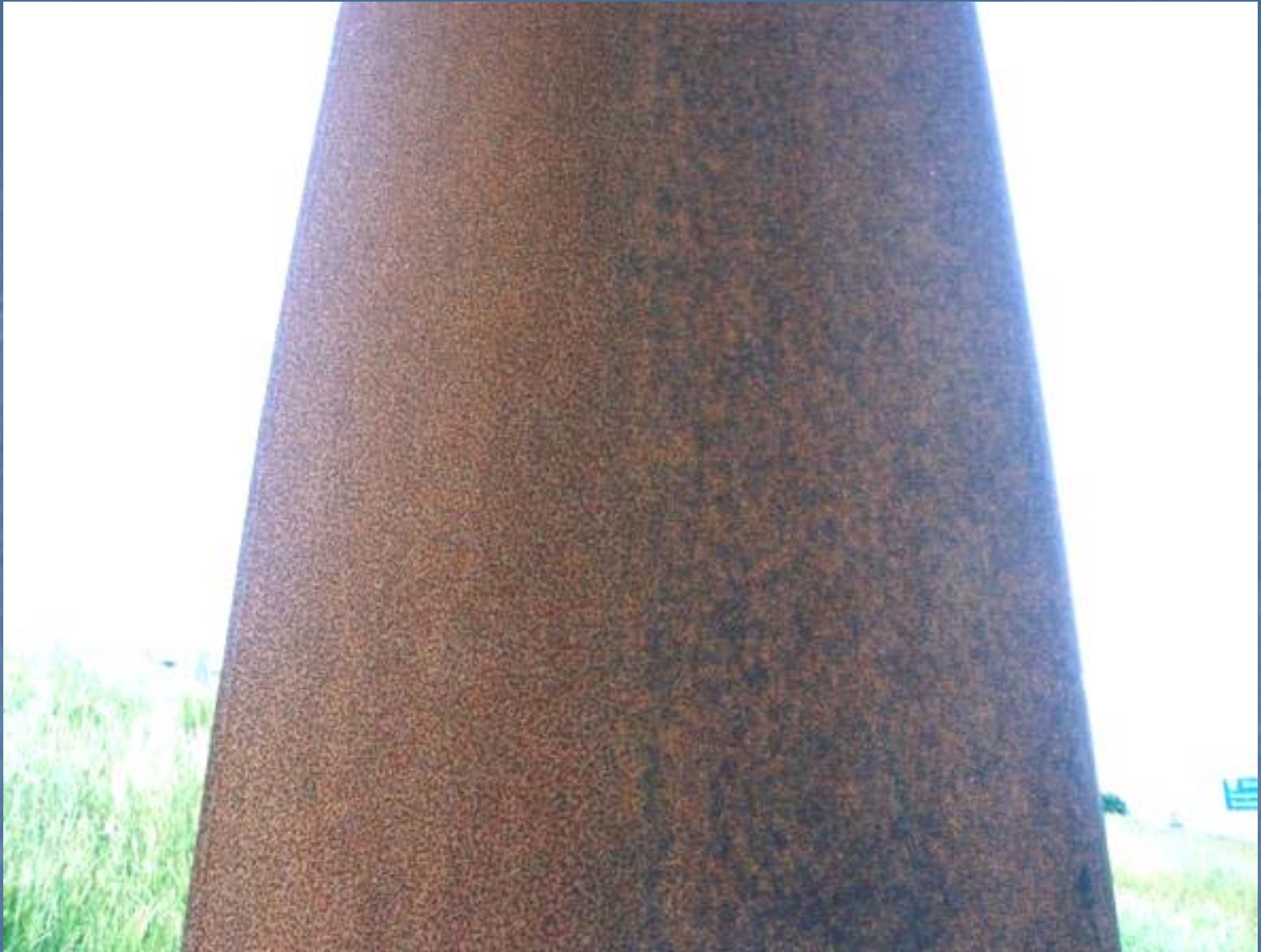
Corrosion Hues on a Weathering Steel
