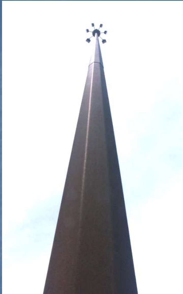
Corrosion on Weathering Steel Lamppost
