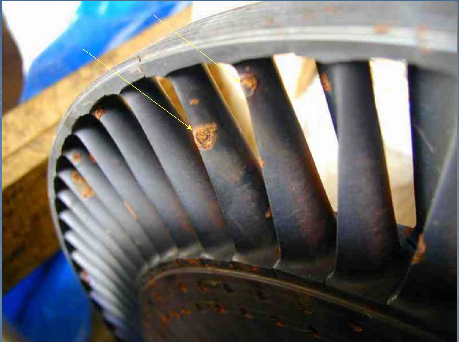
Pitting corrosion of high pressure turbine blades caused by a leaking isolation valve combined with incorrect steam chemistry
