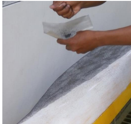
Figure 3. Sticking of sand with wire mesh
