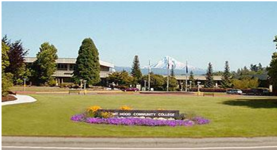
Figure 14. Photograph of Mount Hood Community College Campus, Portland, State of Oregon
