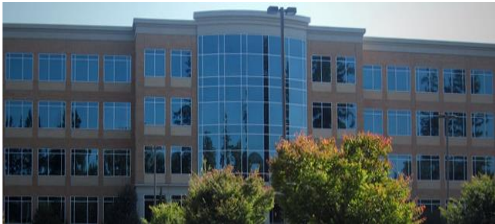
Figure 4. Photograph of The University of Phoenix, Tigard. State of Oregon
