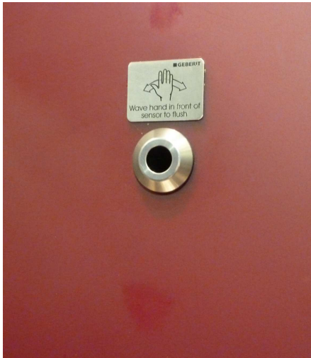
Figure 1. A typical ‘magic eye’ sensor in a WC cubicle in a shared public toilet in the UK. The physical form of the sensor does not follow function hence the presence of the small explanatory sign indicating usage in text and image. The fact that signage is deemed necessary is indicative that these kinds of touch-free sensors are not yet sufficiently common and standardised to be transparent; it is not necessary to sign the usage of a WC push handle flush. (Source: author photograph.)
