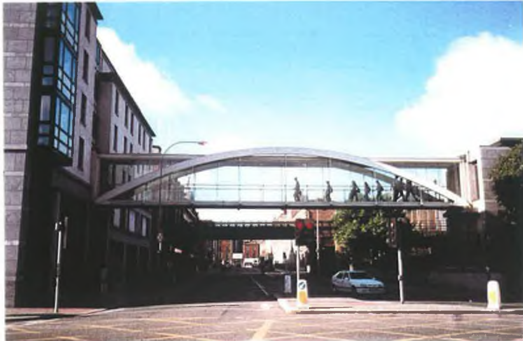
Figure 6: Symbolic Glass Bridge
