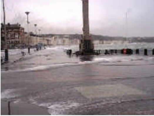
Plate 2.4 Overtopping at the Douglas Promenade.
