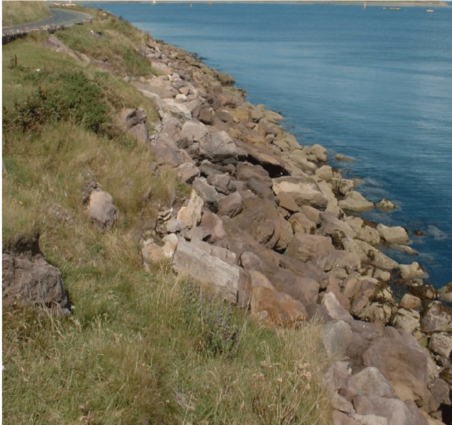
Plate 8.4. Coastal squeeze – protection to prevent further erosion.
