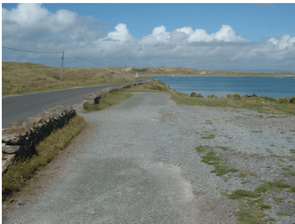
Plate 8.3. Road setback as a consequence of coastal erosion on a soft coastline.
