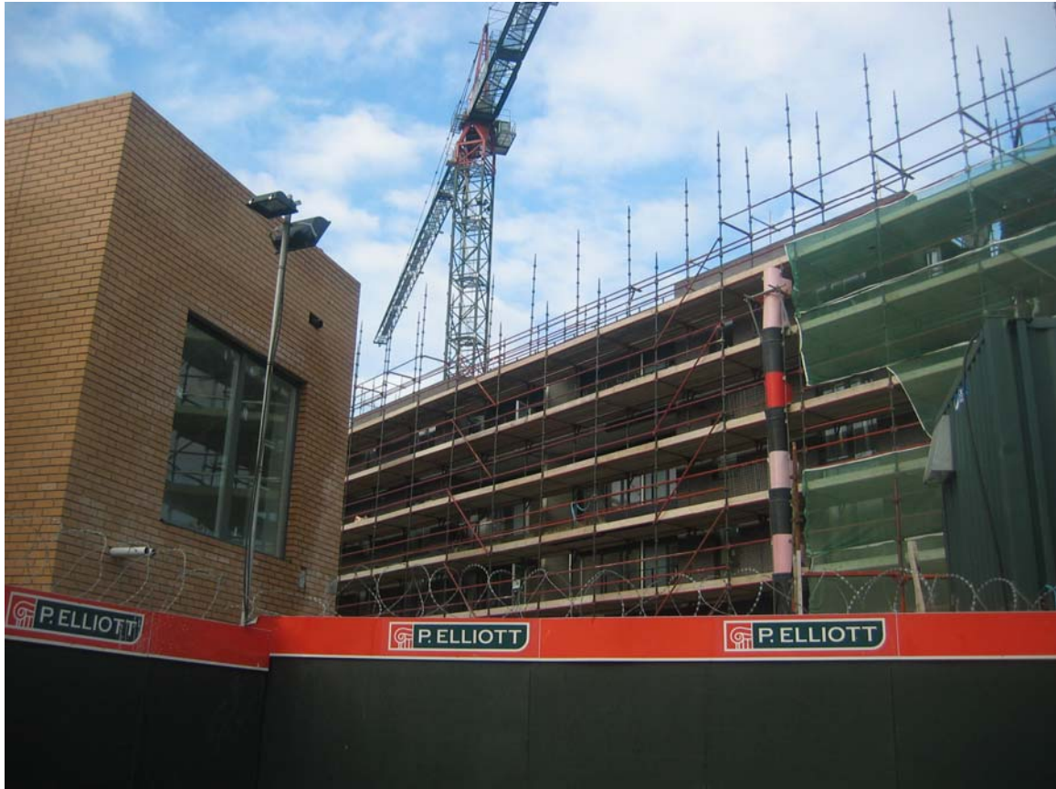
New Fatima under construction, 2008
