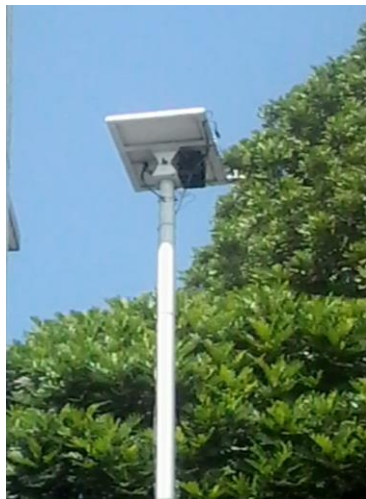
Fig. 5 In situ testing
