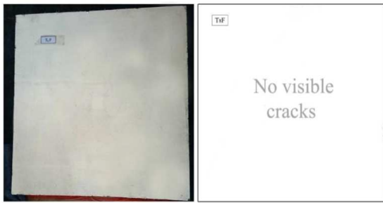
Fig. 7 Crack pattern of the slab T 8 F
