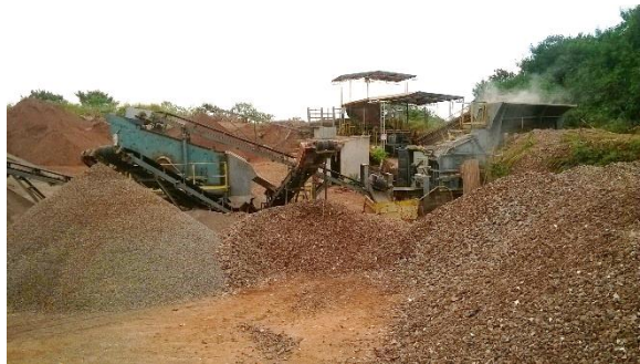
Figure 19. Stationary C&DW recycling facility located in São Paulo State.
