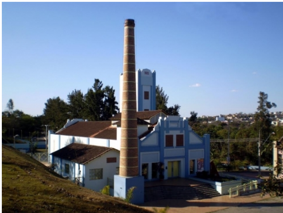
Figure 1.1: The Gravatá Mill in Divinópolis SOURCE: (DIVINÓPOLIS, 2017).
