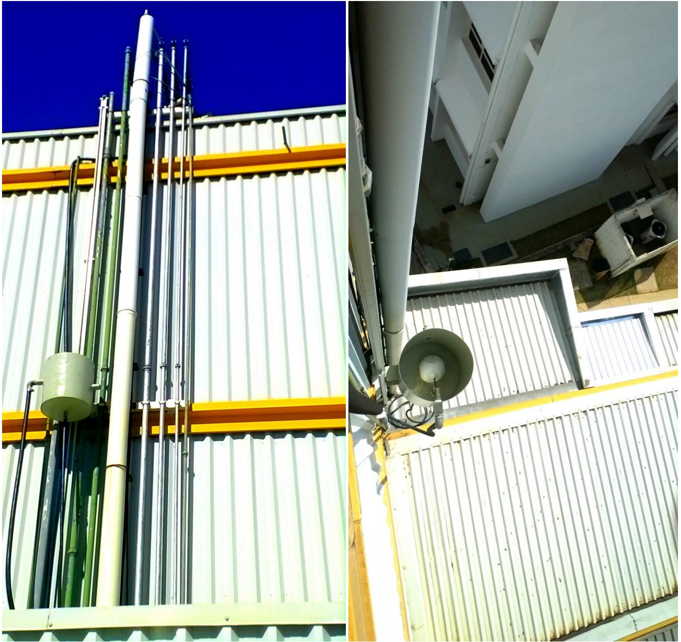
Figure A. 5– Photograph of the vertical section side and top view
