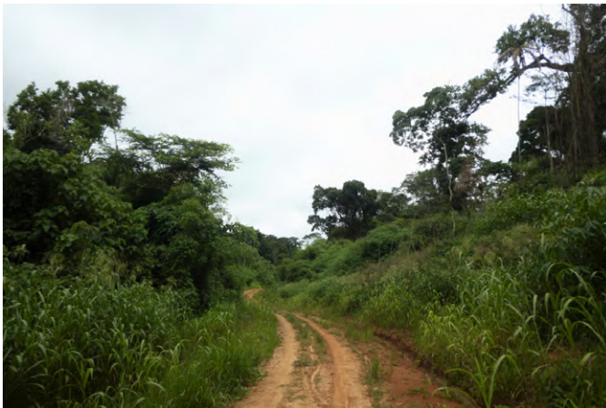
Figure 2. General view of the Riozinho do Rola road, Rio Branco, Acre State. Photo by COAG.
