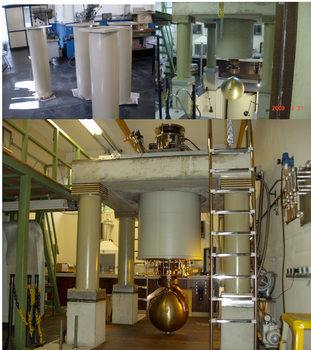
Figure 7. In order to immobilize the sphere cryostat at a high position (about 1.5 meters up), large tubes were constructed as “columns” for the detector concrete base, bringing the antenna to the floor level. A wood floor was constructed under it, making the transducer assembly work easier. Two “swimming pool” ladders were installed for access to the top of the detector.
