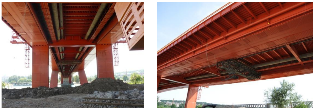
Figure 3.1: Tested part of GAZELA Bridge for AVM
