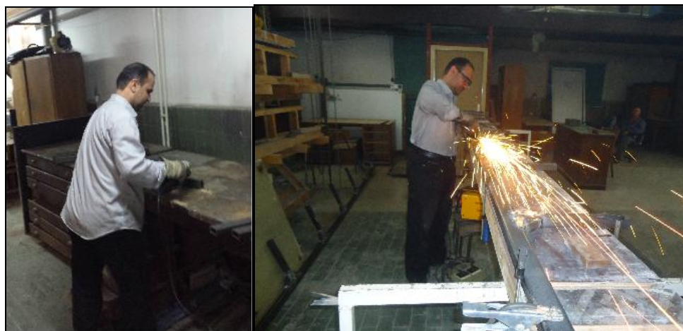
Figure 5.18: Preparing the main steel sections of the grid-bridge model
