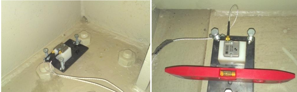
Figure 3.2: Accelerometers handling and installation in test of structure of GAZELA bridge
