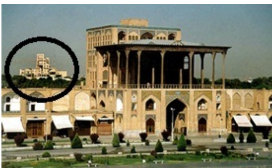
Figure 1: Naghsh e Jahan Square in Isfahan (Jahannama Tower)
