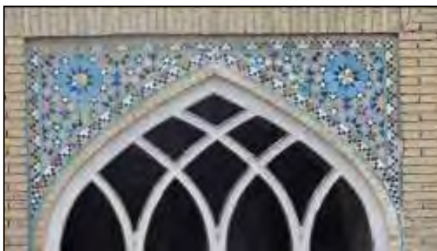
Figure 13. A gere accomplished in a form of spandrel
