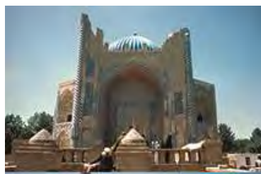
Figure 9. Khwaja Abu Nasr Parsa shrine (view from northeast, vault and entrance part )
