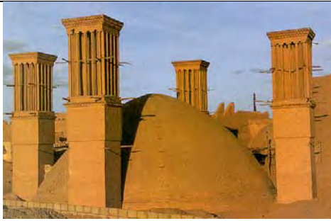
Figure 9: Reservoir with six wind tower
