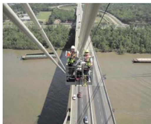
Fig 2. Cable inspection with hanging lift.
