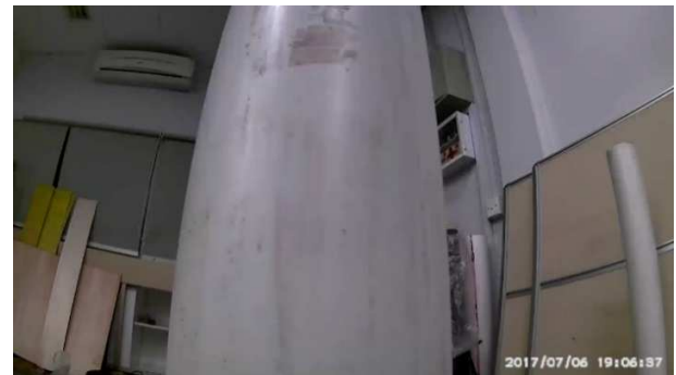
Fig 9. Captured inspection image from camera
