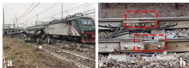
Figure 1. Pioltello (Mi, Italy). (a) Train accident; (b) Rail point where the failure may have occurred [2, 3]
