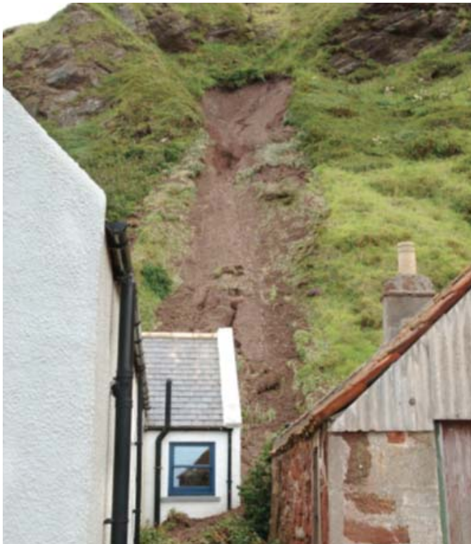
A property is partially buried by a mudslide in Pennan, Aberdeenshire, August 2007. Image ©NERC
