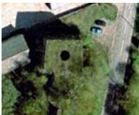
Figure 13. Google Earth image of the draw line at the Derry Lime Works at Cults (eastern Scotland). Note the massive square masonry structure surrounding and supporting the kiln (the central circular feature).
