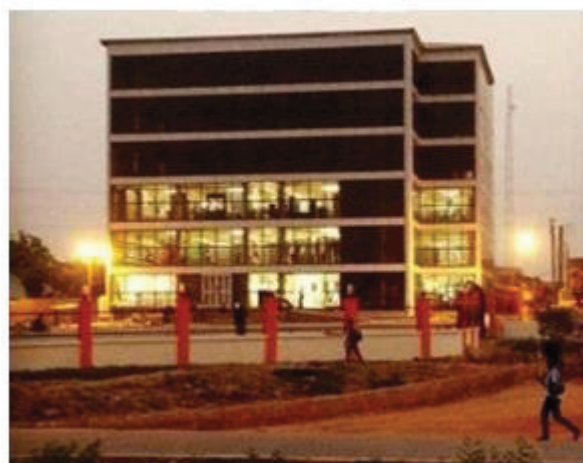
External View before Collapse
