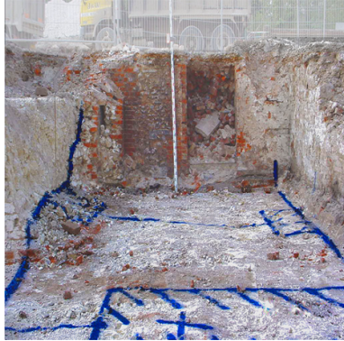
Fig 1 Mitchell Bould, Setting out of Osborne School onto a Victorian Cellar. Setting out drawing by Fred Rees, Site Engineer, Photograph by Dan Keeler, Architect, represented at the Winchester Gallery 2004.
